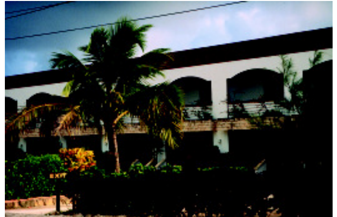
Here in the Marianas we often employ the familiar red tile roof and plastered white or simulated adobe-brick walls.
