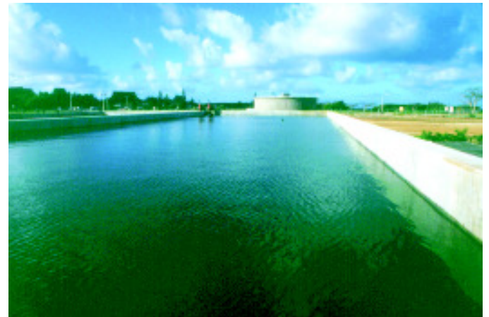
Effluent from our sewage treatment plants is piped directly into ocean water. Currents disperse Saipan's two outfalls' wastewater around our lagoon and nearshore waters.
