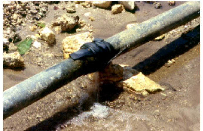
Leaks in our water pipes need to be repaired properly. Temporary control measures can lead to significant water loss.
