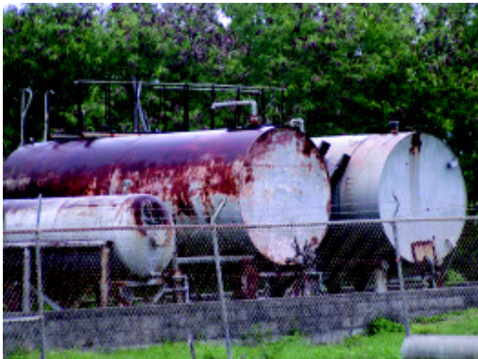
When tanks, piping and transfer equipment are poorly maintained, or improperly used, spills and leaks can occur.
