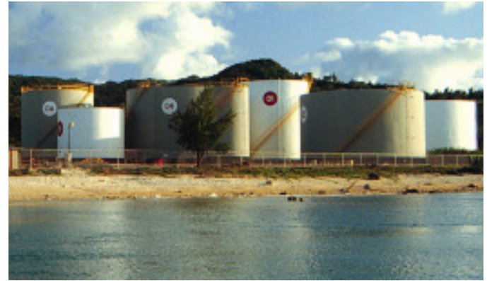
Fuel tank farms located at harbor sites are a major source of potential water pollution that few people recognize.
