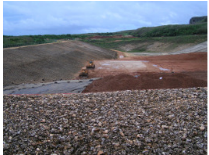
RCRA establishes guidelines which ensure that standards for the design of landfills are implemented correctly. Saipan's Marpi landfill meets these standards.
