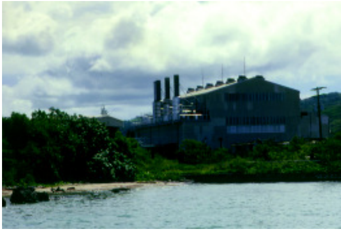
Diesel engine generator units produce Saipan's, Tinian's and Rota's electricity.
