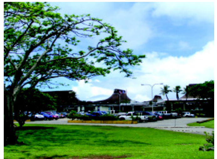
The Francisco C. Ada Saipan International Airport is the largest airport in the CNMI.
