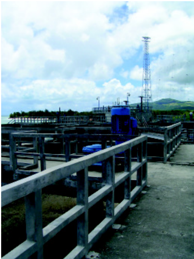
The treatment plant is designed to process large quantities of wastewater on a continual basis.
