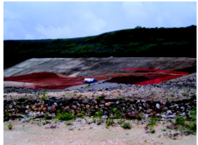
...it is then covered with an adequate layer of soil at the end of each day.
